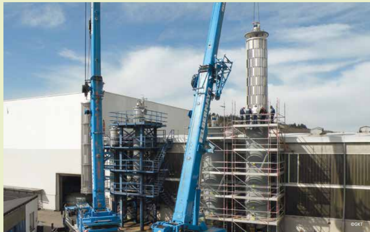
Assembly of a short-path evaporator
