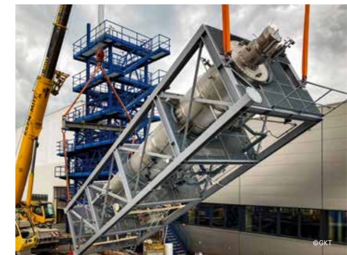
Thin-film evaporator – skid unit
